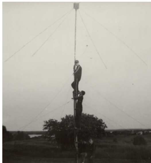
Installation of the Square for 10- 15- 20- meters
