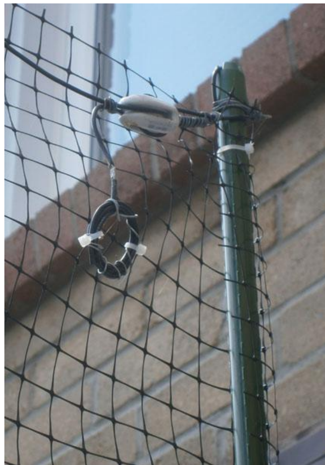
Photo 6 Roll of wires in horizontal wire
