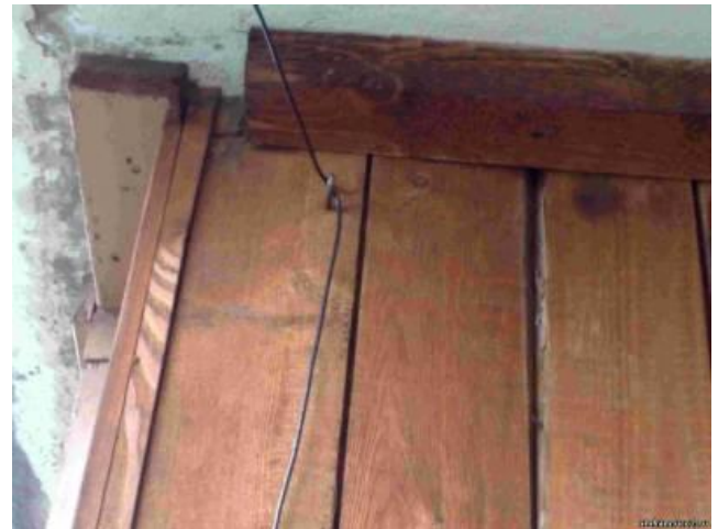
Picture 2 Nails for Fixing the Loop Antenna
