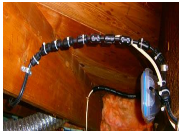
Figure 2 Ferrite Clips on the Coaxial Cable
